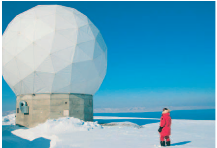
Figure 2. The radome housing the 11m antenna for NASA support
