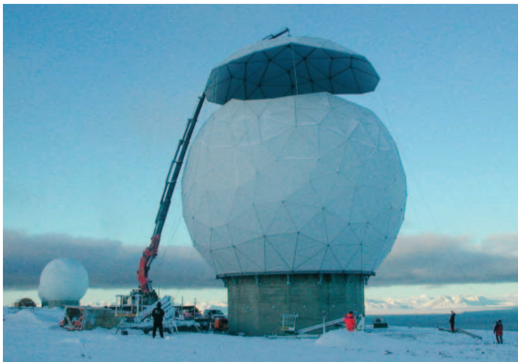
Figure 4. Installation of the radome for the new 13 m antenna
