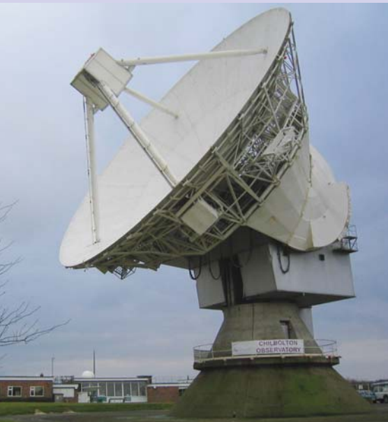
The Chilbolton S-band radar of RAL at Chilbolton, UK (RAL)
