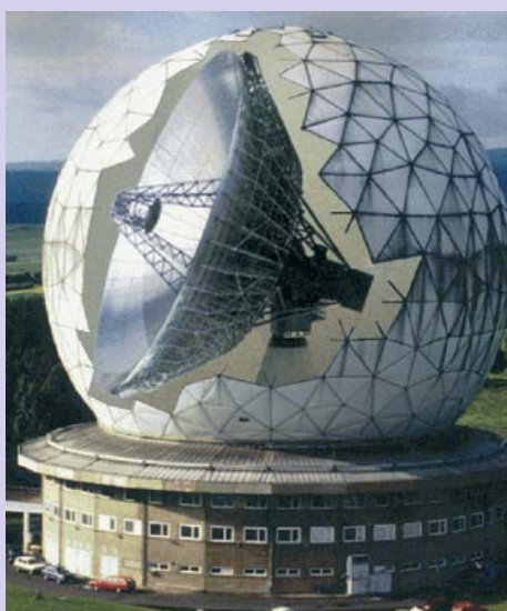
The TIRA L and Ku-band radar of FGAN at Wachtberg, Germany (FGAN)
