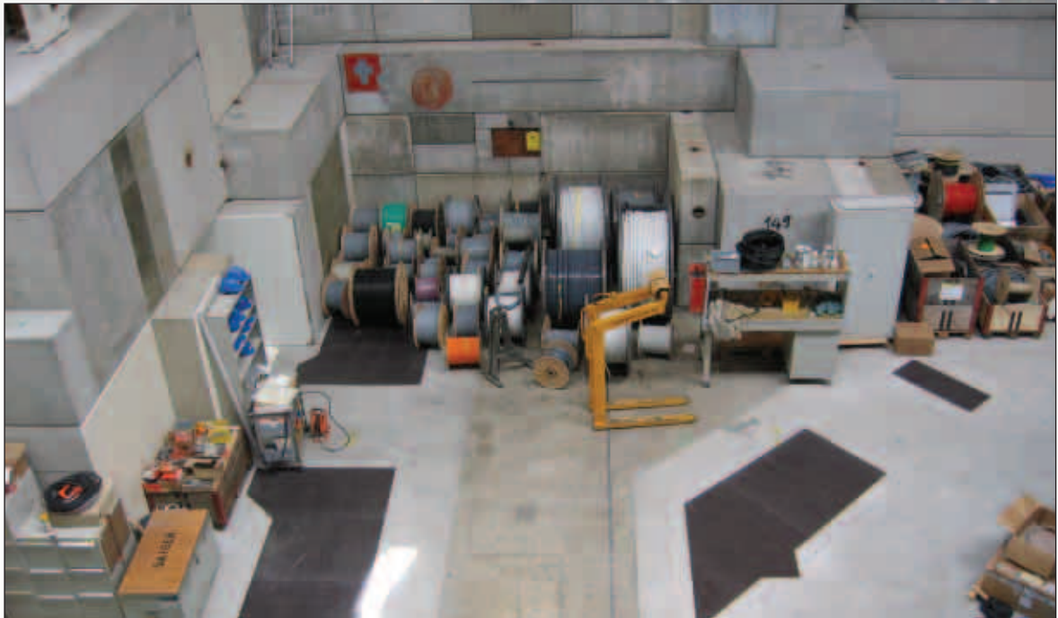
Future PIF Area Under Construction
