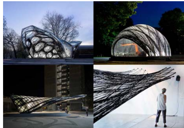
Fig. 2. Precedent examples of fibrous based fabrication methods for differentiated and lightweight structures. From upper left, clockwise. ICD/ITKE Research Pavilion 2013/2014. ICD/ITKE Research Pavilion 2014/2015, Mobile Robotic Fabrication Eco-System by Maria Yablonina of ICD, ICD/ITKE Research Pavilion 2016/2017.
