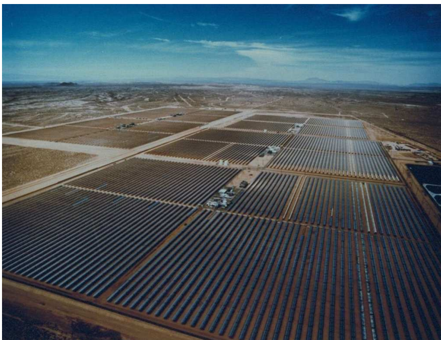
Figure 46. Solar Thermal Trough Power Plant in Kramer Junction, USA
