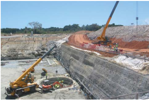
Excavation of the large Russian-style flame duct for the new Soyuz Launch Complex (ELS) at Europe's Spaceport in Kourou (Fr. Guiana) in March (Photo: ESA/CNES - Photo Optique Video CSG)
