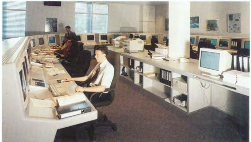
Cluster Dedicated Control Room
