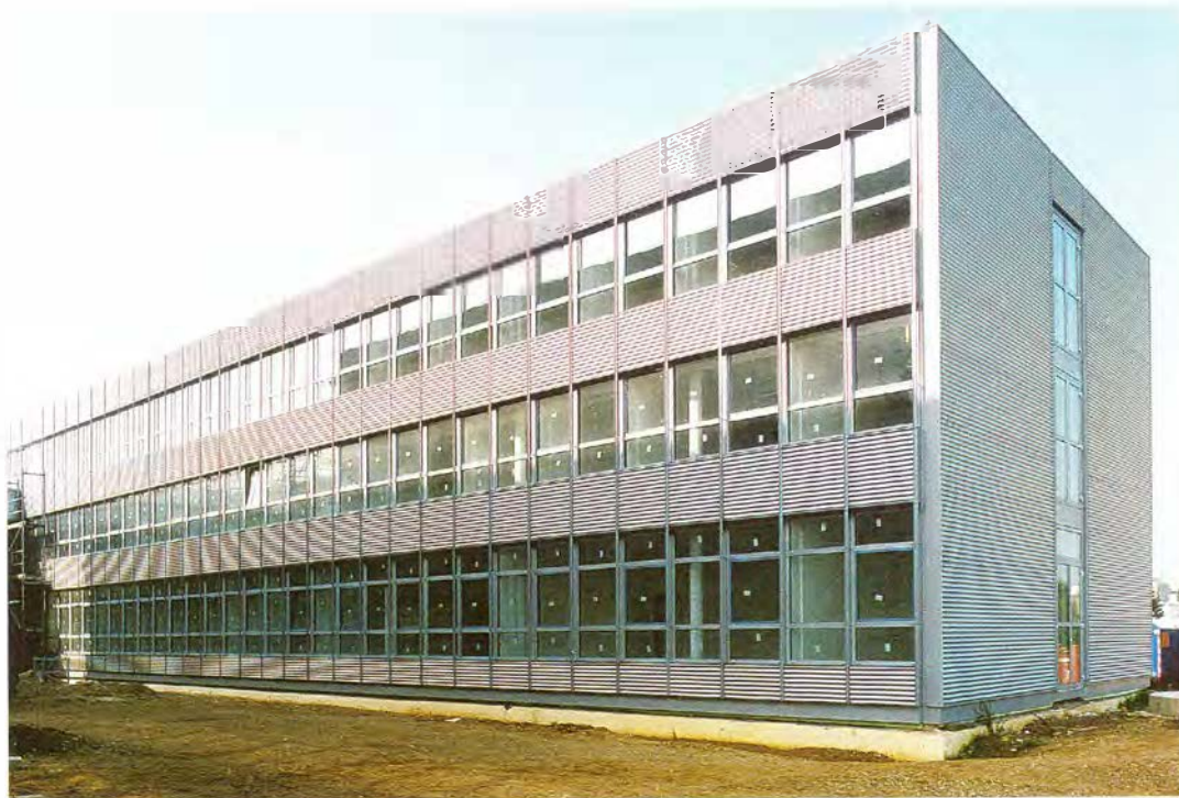
Figure 4. New EAC accommodation: the Crew Training Complex
