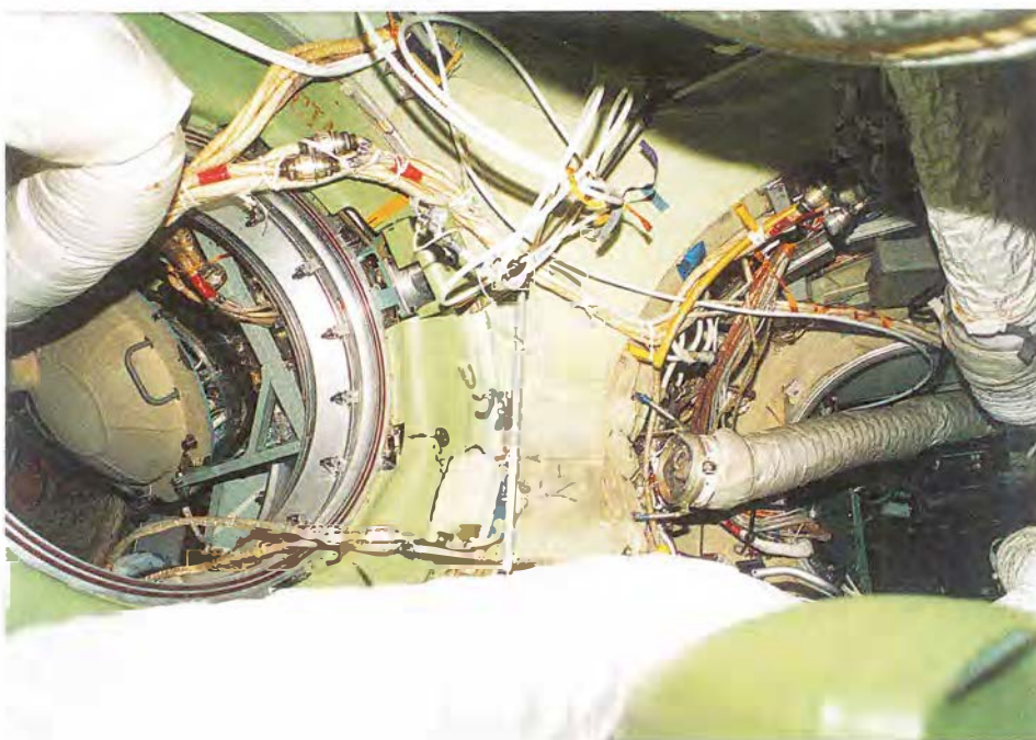
Figure 3. Some of Mir's flexible ventilation ducting
