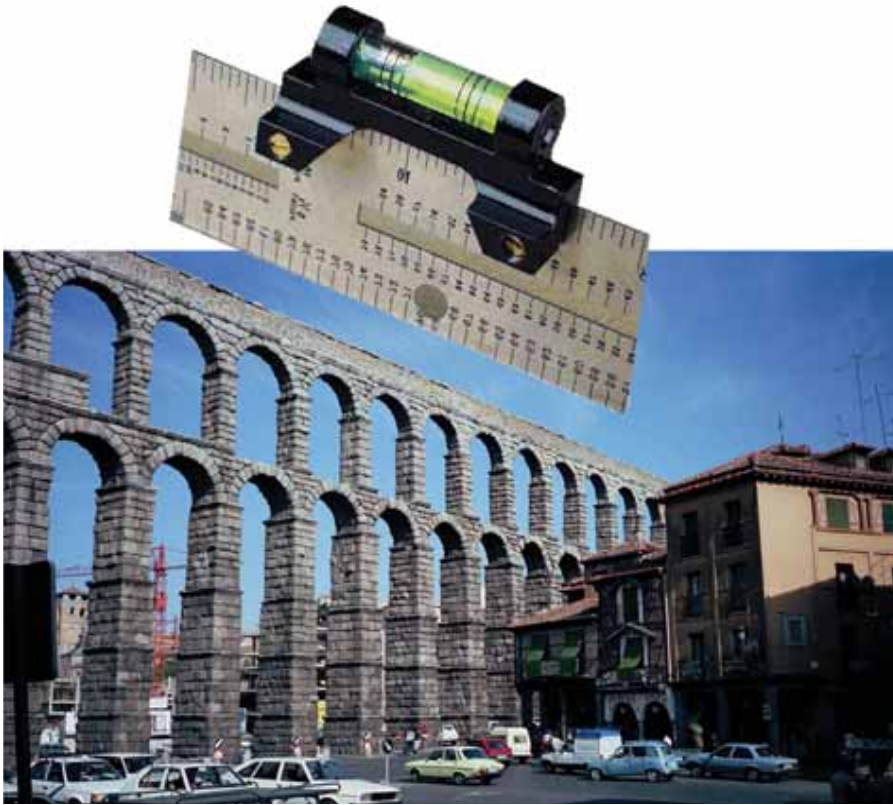
Modern local surveying tools, such as the spirit-level, simplify levelling on a small scale. But construction of early water-bearing structures, such as Roman aqueducts, relied on traditional levelling methods to transport water
