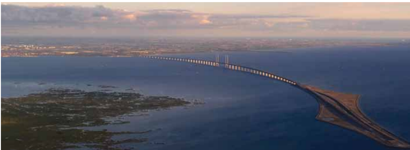
The Øresund bridge and tunnel system between Denmark and Sweden connected two national height systems
